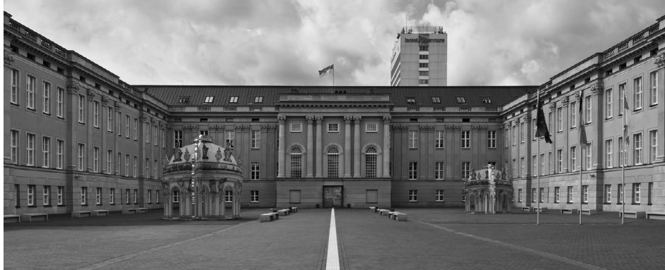
The public inner courtyard.
