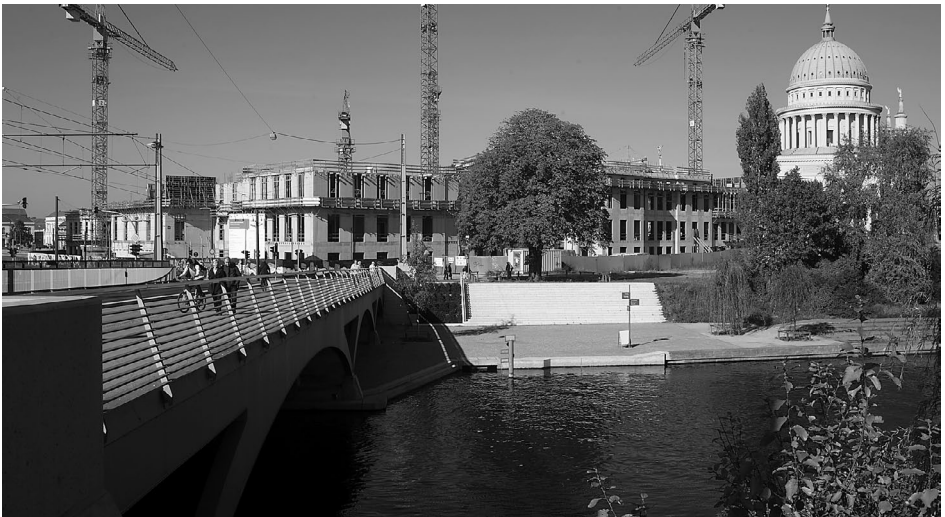
View of the construction site for the new Landtag building.
